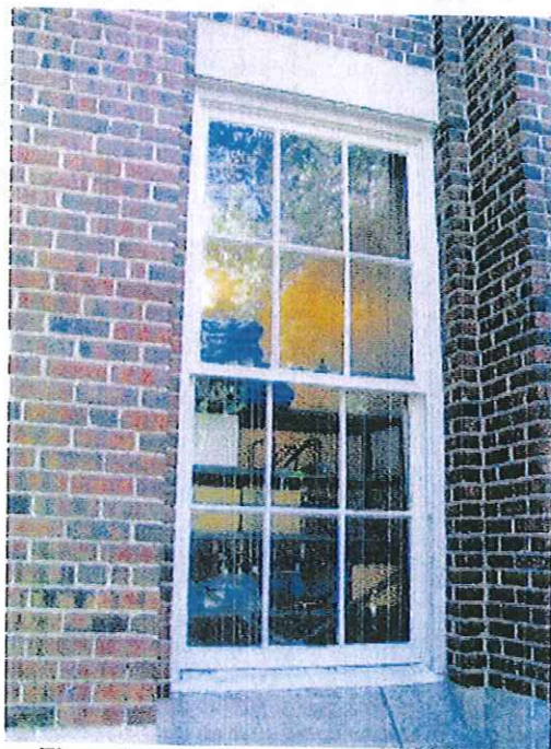
Figure 128: Exterior view of window type D.
