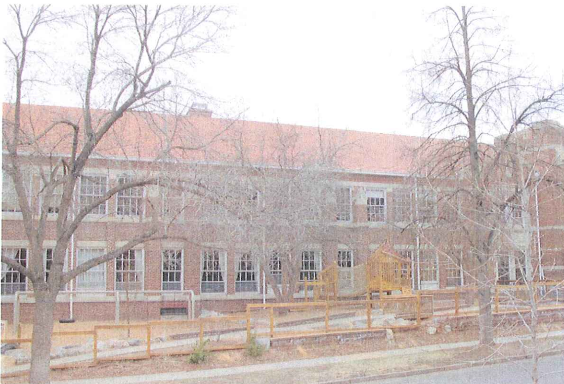
West Elevation on Fillmore Street
