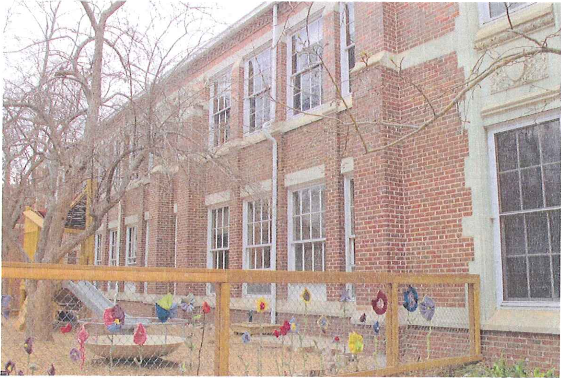
West Elevation - Kindergarten Playground
